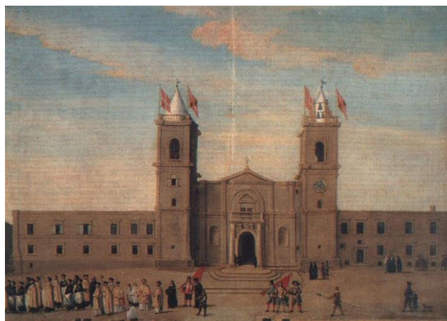
Dedication of the Principal Church of the Order, Conventual Church of Saint John the Baptist, in Malta
